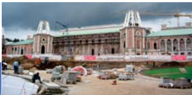
The course of the restoration
